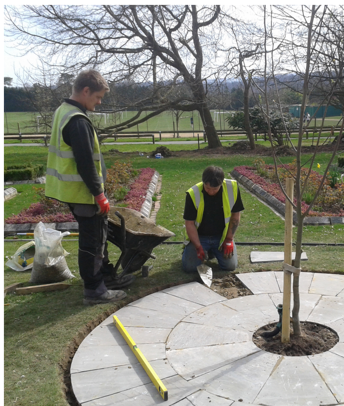
DS Restoration paving at the Lower Rose Garden
