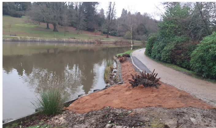
Repairs to lake banks and path, December 2019
