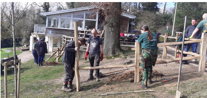
Monday Volunteers installing protective fence around Cafe Oak, March 2020
